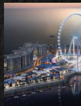
Bluewaters Island Dubai United Arab Emirates
