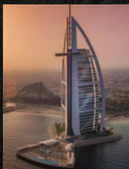
Burj al-Arab Abu Dhabi United Arab Emirates
